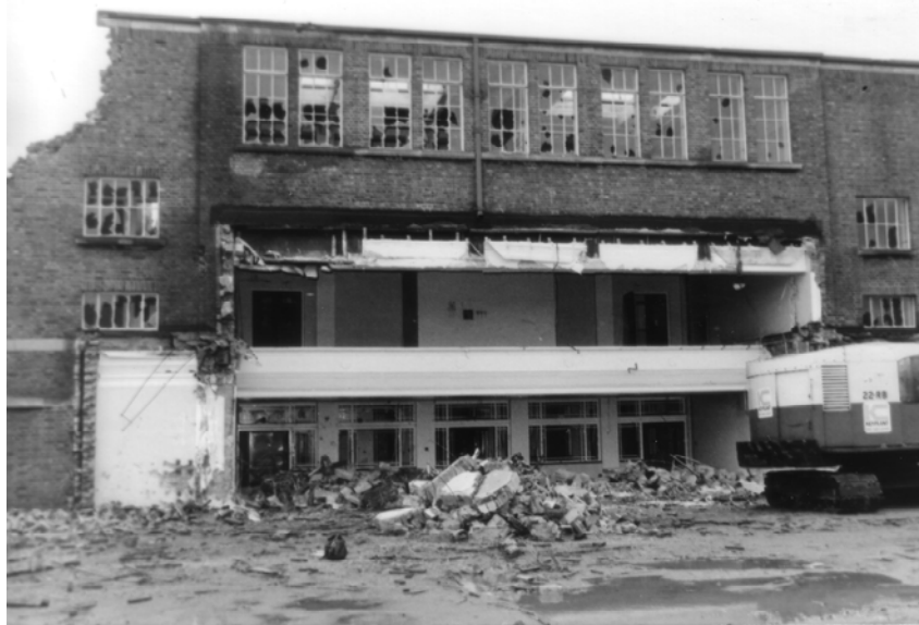
The reverse view, from what used to be the school hall, looking towards the front corridors.
