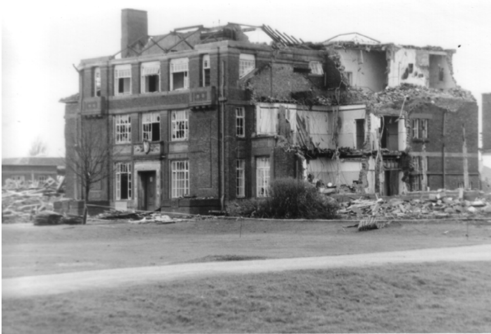
The final centre section of the main building
