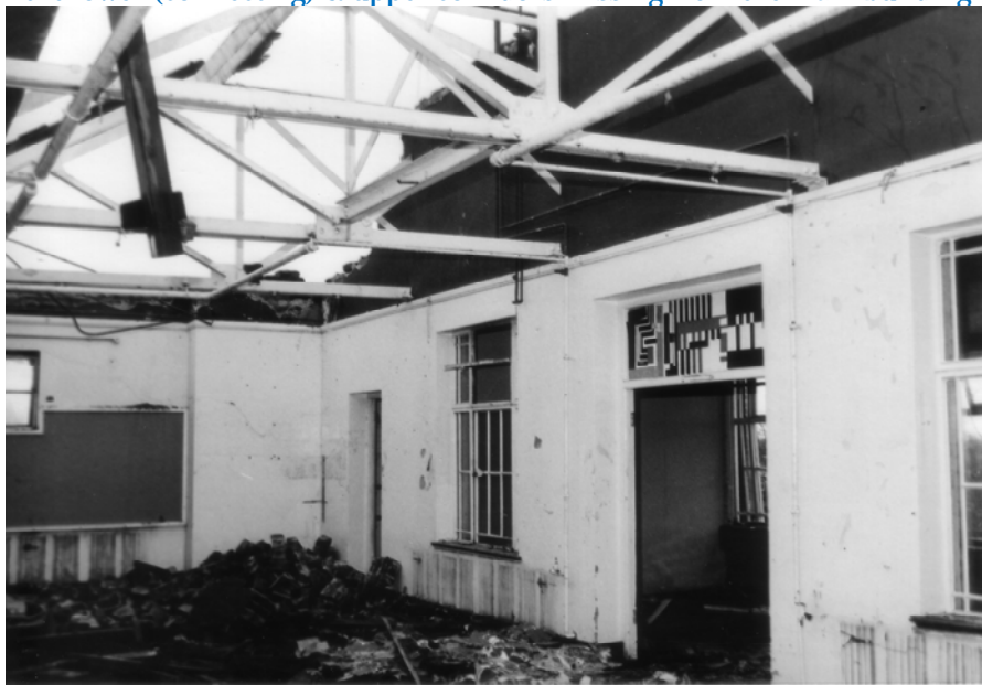
The art and music rooms on the 2nd floor in the main building
