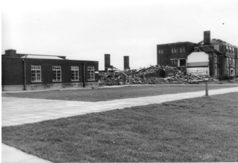
(From the main road), the Wood/Metal Work room in the foreground, with the lower (connecting) & upper corridors missing from the main building
