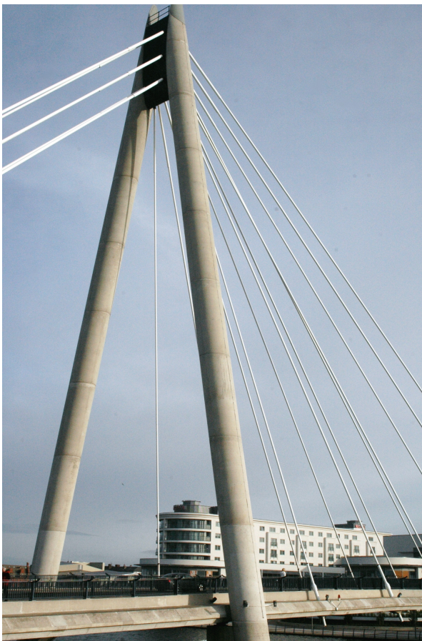
The Marine Way Bridge
