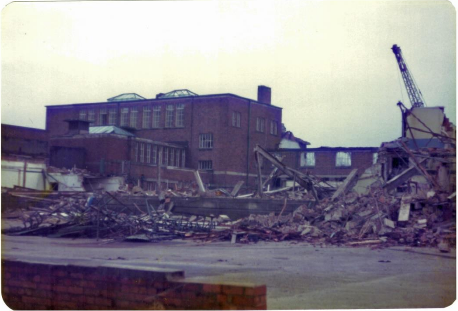
The centre section of the school, from the North West area. The space behind the low wall used to be occupied by the changing rooms
