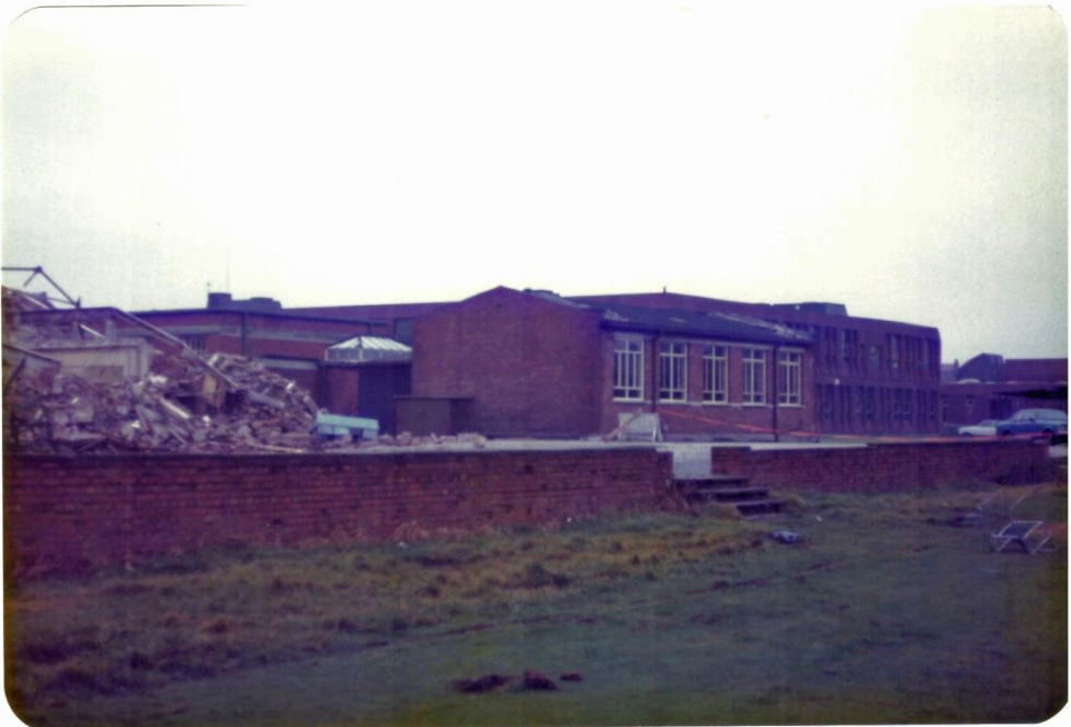
The Chemistry Lab at the rear of the school, with the new College building in the back ground. The steps leading down to the field were behind the demolished (left of picture) changing rooms.
