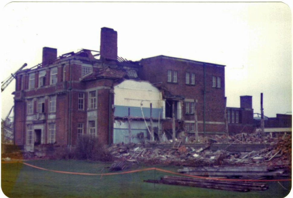
The centre section of the school, from the East wing
